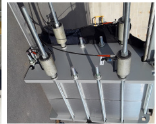
THS SERVICE DISASSEMBLING PHE
