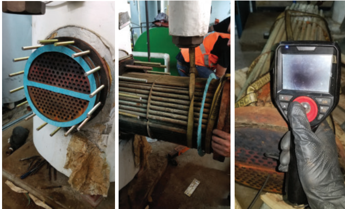
CUSTOM ONSITE GASKET FABRICATION, BUNDLE REMOVAL & INSTALLTION, BORESCOPE TESTING
