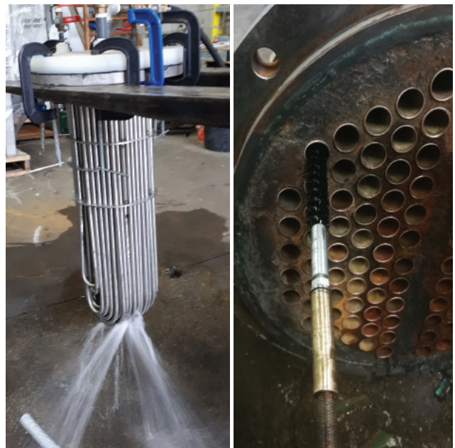
SHELL & TUBE PRESSURE TESTING
