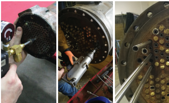
TUBE VACUUM TESTING, CLEANING, REPLACEMENT, TUBE PLUGGING, SLEEVING AND EXPANDING
